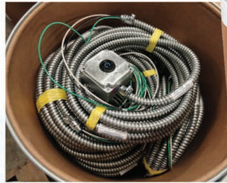
Cables placed in a barrel
